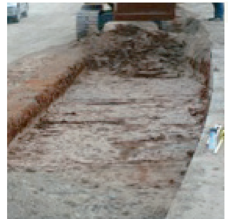
Figure 1. Removal of old pavement and boxing out for new Bitumix pavement
