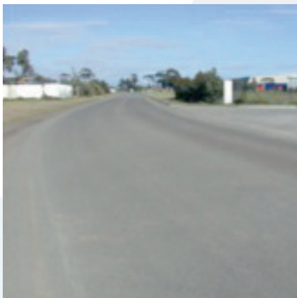
Figure 4. Completion after 12 months prior to hot mix wearing course placement
